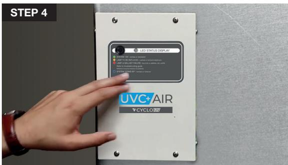
4. From now on, the UVC+ AIR will only activate the lamp when the thermistor detects airflow in your duct system.
