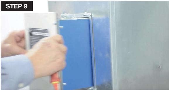
9. Once the new UV lamp is installed, replace the UVC+ AIR into duct. Then, reset your product and its lamp timer (see page 9).
