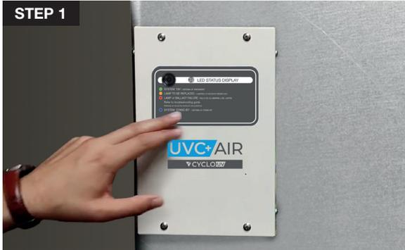
1. To reset the lamp timer the unit needs to be powered and turned ON. The status LED should either be "Green" or "Blue" (heartbeat).
