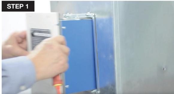
1. Take the UVC+ AIR out from the ductwork by removing the 4 screws located on the cover (4 corners) that hold it to the frame.
