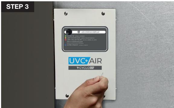
3. Press and hold the reset button for a minimum of 3 seconds. When releasing the reset button, the counter will be reset to 1096 days.
