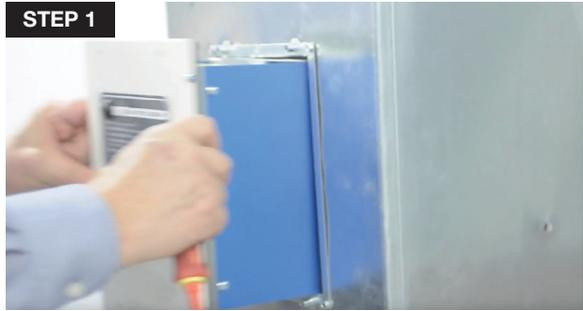
1. Take the UVC+ AIR out from the ductwork by removing the 4 screws located on the cover (4 corners) that hold it to the frame.
