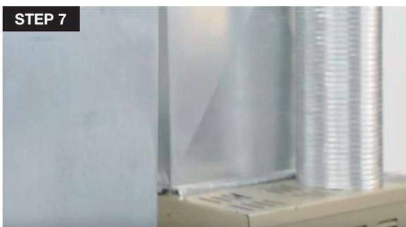
7. Prepare the duct (return or supply) for installation. Evaluate the ideal area for installing the air purifier. The reflection chamber should always be parallel to the airflow. Ensure that the purifier will fit into the plenum and position it keeping in mind to minimize plastic exposure to direct UV light.
